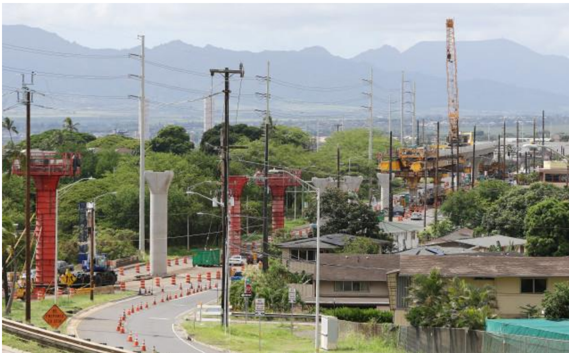
The rail project was under construction near Aiea in late September.
